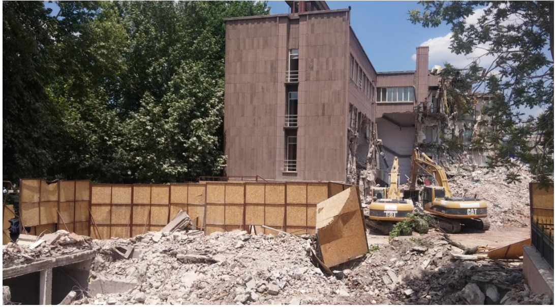
Figure 4.19. The demolition of İller Bankası (Source: http://www.mimarlarodasiankara.org/download/İllerBankasiDurumRaporu.pdf )
